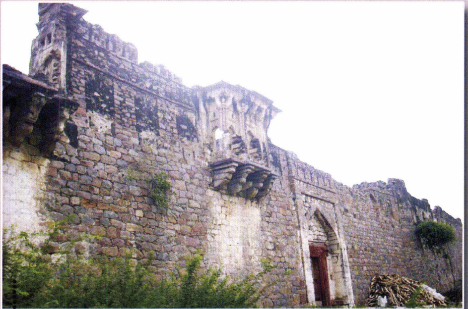
● A side view of the Fort, Devdurga Fort, Raichur Dist .
